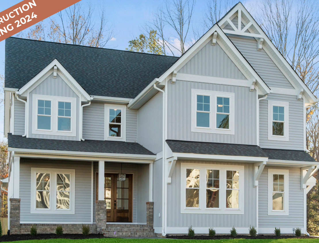
Representative photo. Home under construction.
